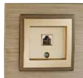
prise telephone (RJ11 Cat3)
